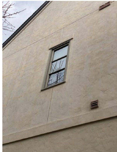
Vent not sealed properly
