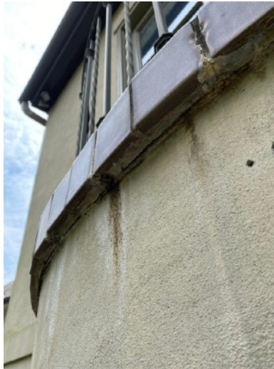
Missed drip edge flashing
